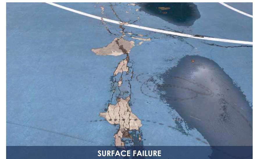
PATCH WORK AND SURFACE FAILURE, PUDDLING
