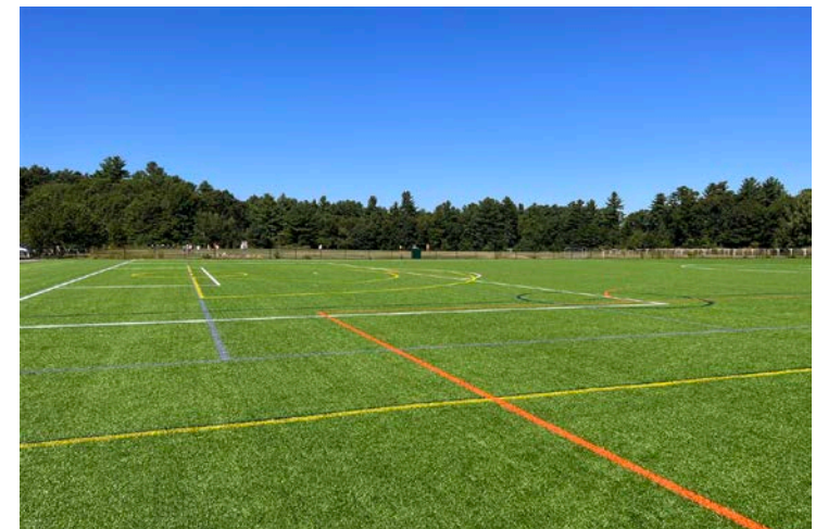
Infill Installation and Final Grooming
