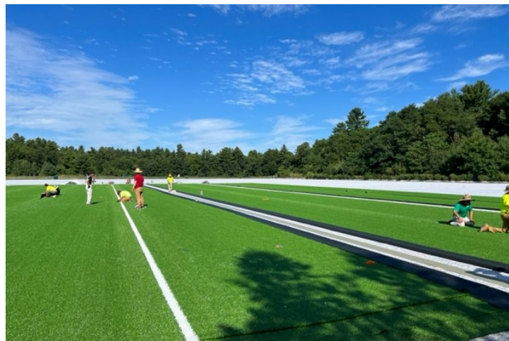
Installation of Turf and Inlaid Markings
