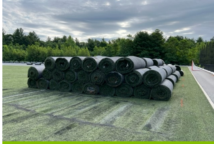
Removal of Existing Turf and Infill
