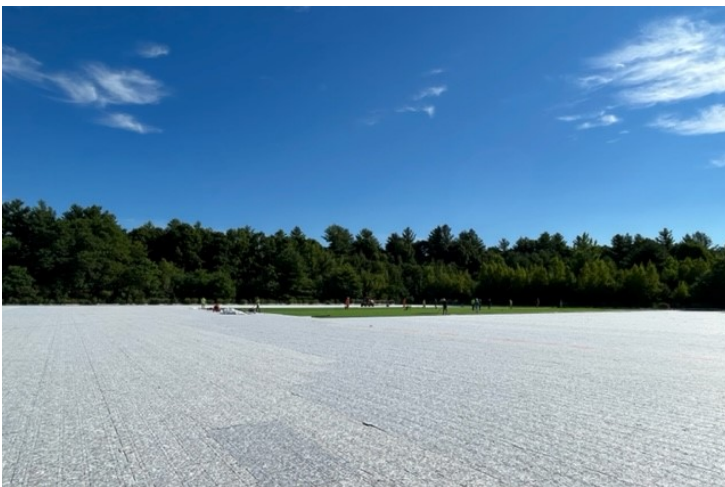
Installation of Shock Pad (if required)
