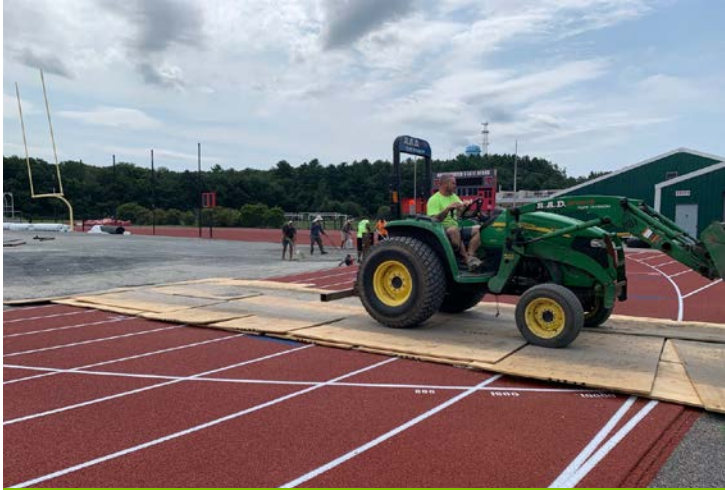
Protection and Erosion Controls
