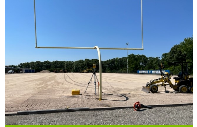
Laser Grading of Stone Base
