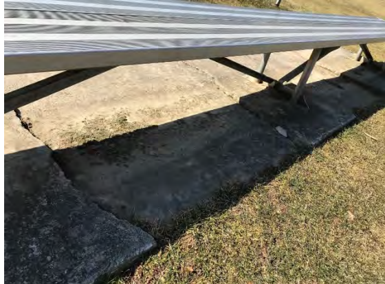
Wet infield. Bowed mesh and cracking concrete bends under player's benches.
