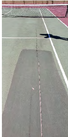
Cracking surface and fading sealant.
