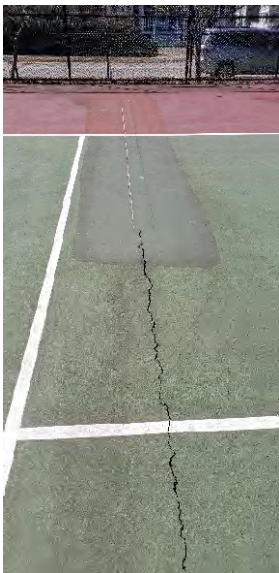
Cracking surface and fading sealant.
