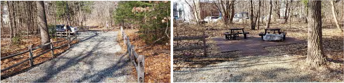
Off-street parking with picnic area. Space for approximately 3-4 vehicles. Two (2) Uline picnic tables on composite decking with ramp. One accessible picnic table.
