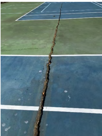
Heavy, hazardous cracking across court surface but particularly in field of play. Fading sealant.
