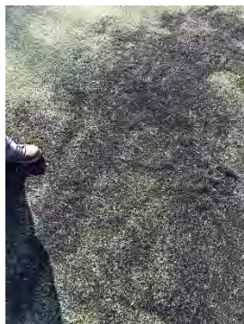
Some concrete, fencing, turf fibers and other elements in need of repair or regularly scheduled seasonal maintenance.
