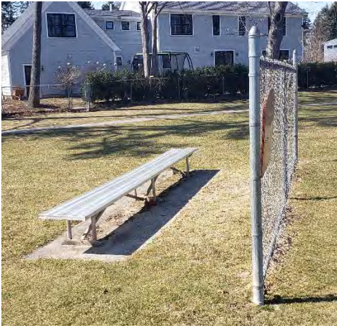
Mesh bowed at backstop.
