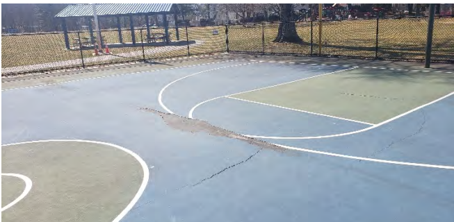
Cracking and fading of sealant on both courts.
