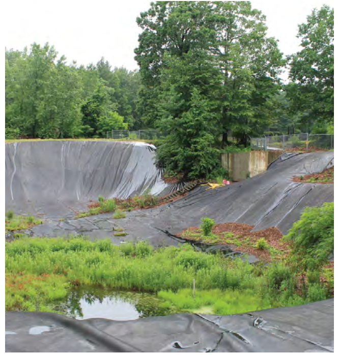
Existing basin (with capped contaminated soil).
